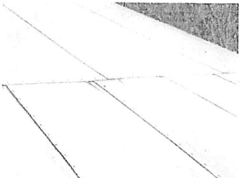
Roof exterior: showing roof lap seams to be generally tight with no open penetrations observed.
